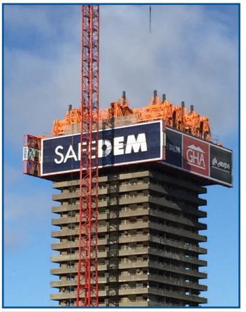
We are gearing up for the arrival of the TopDownWay® System at 120 Wyndford Road. This is an innovative modular system whose shape can be adapted to that of any high rise structure to be demolished.
