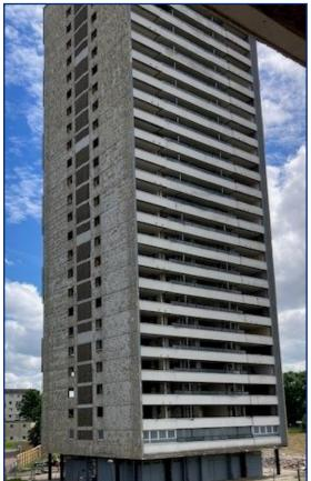
All 4 buildings have been 99% stripped of fixtures and fittings and any hazardous materials removed. So far, we have removed 1,850 tonnes of waste, with 99% of this waste being diverted from landfill, for re-use primarily within the construction industry. All asbestos has been safely removed from all 4 buildings, following all strict health and safety guidelines.
